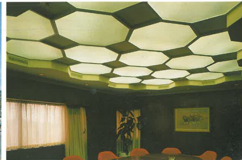
BELOW: The versatility of fibrous plaster is illustrated in this ceiling effect created in the boardroom of a modern office block in Wellington. Tiles for the ceiling were made to specification by Plastercraft Industries Ltd.
