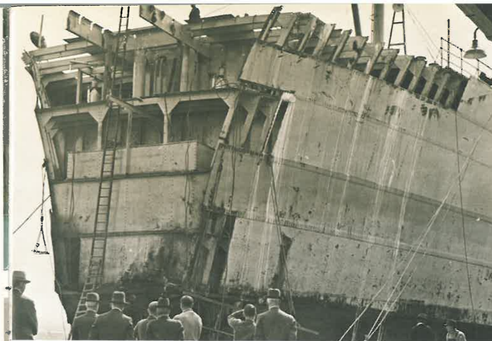
ABOVE: The sight of the Norwegian tanker Ole Jacob with her bow missing stopped many passers-by on the Auckland waterfront in 1940. Mason Bros rebuilt the bow section in just over seven weeks, working entirely without plans.
