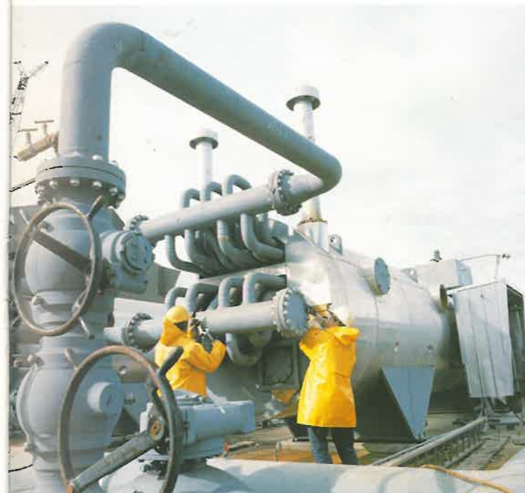
BELOW: The massive Huntly power station complex on the Waikato River near Hamilton is providing on-going contracts for a number of Ceramco subsidiaries. Refractories, ceramic tiles, special industrial linings and piping have been installed, together with cranes, winches, boilers and these large vessels (above), which will pre-heat natural gas for combustion in the main boilers.
