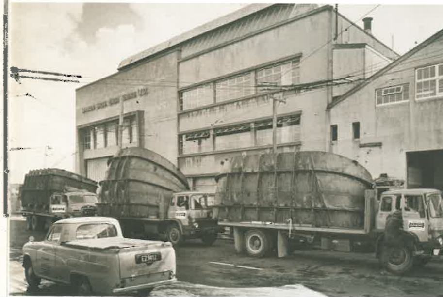
ABOVE: Sections of draft tube liner for the Manapouri power project leaving the Pakenham Street works of Mason Bros Engineering Ltd in 1965.
